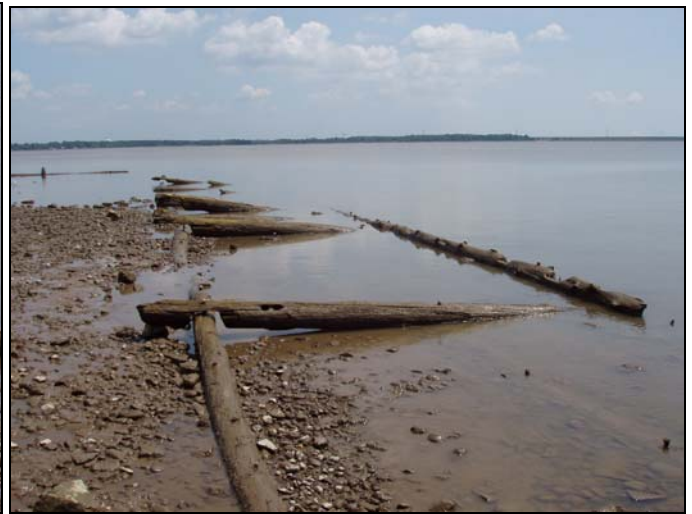
Figure 39. Another view of wooden cribbing
