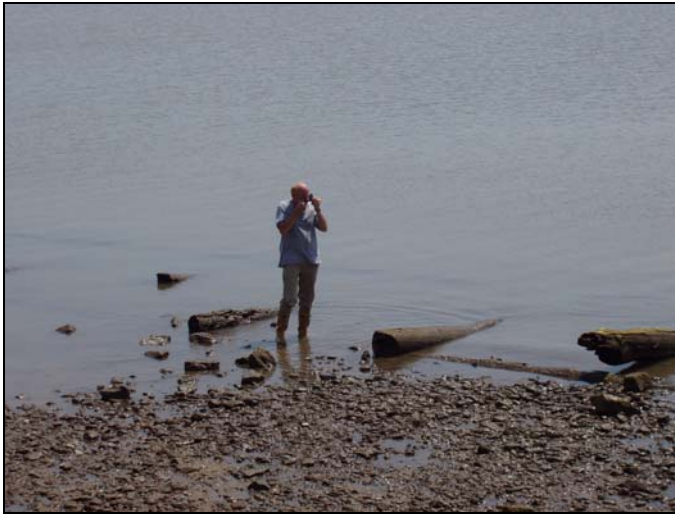
Figure 38. Edge of wooden cribbing and gravel surface.
