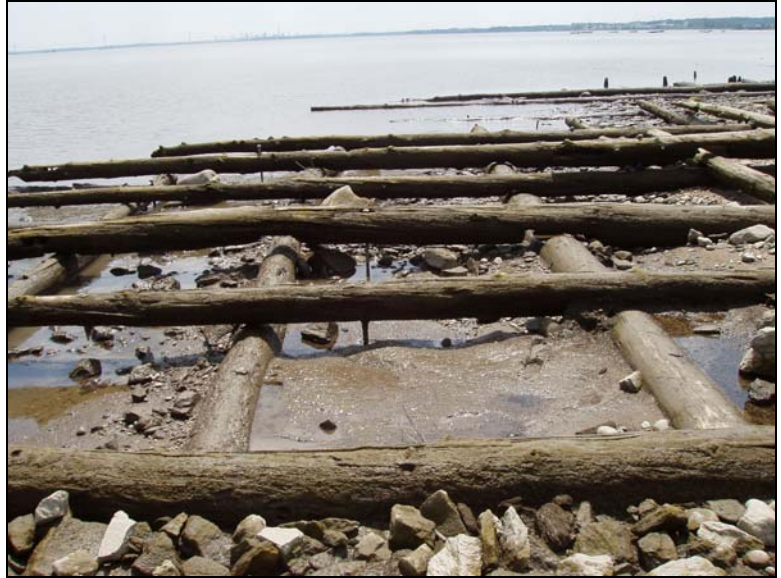
Figure 45. Detail of stacked timbers in cribbing
