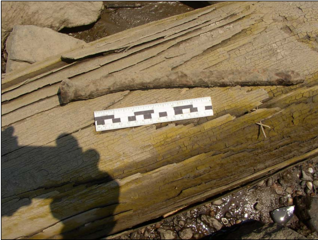
Figure 33. A foot-long spike dislodged from the horizontal timbers along the shore side of the pilings. The head of this spike is pyramidal, as seen in Figure 34.
