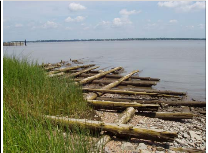
Figure 41. Cribbing viewed to the north. Ice pier F to left.
