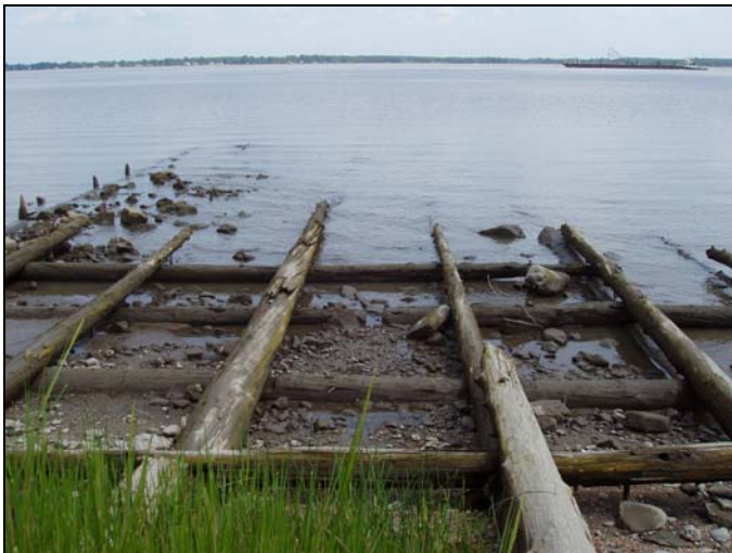
Figure 42. Cribbing further exposed.
