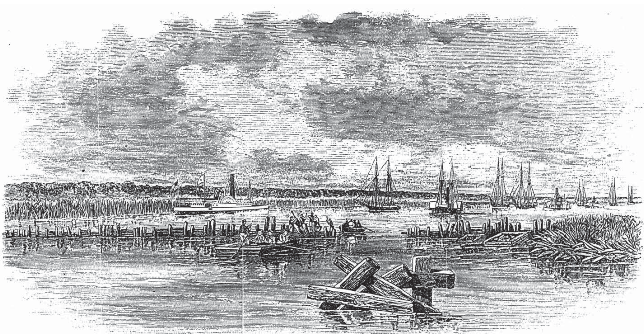
REMOVING THE OBSTRUCTIONS IN THE SOUTH CHANNEL OF THE SAVANNAH RIVER, GA., BELOW FORT JACKSON.
