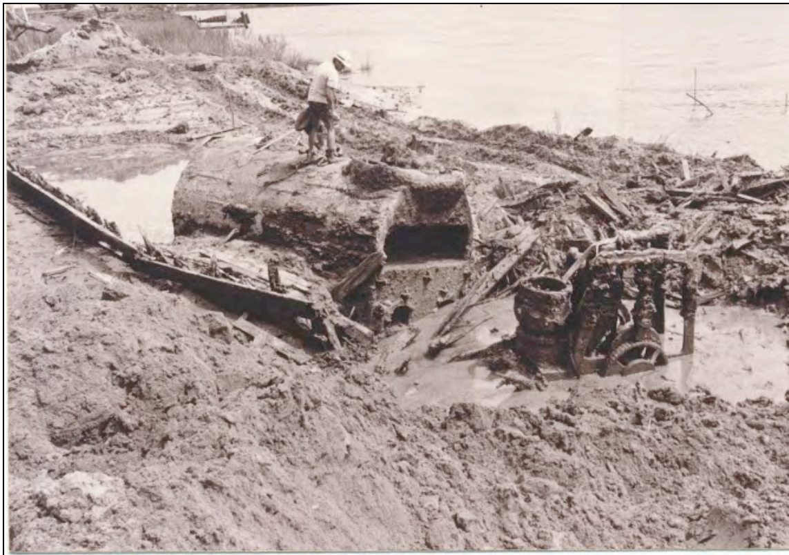
Figure 58. Photograph of Savannah/Fig Island tug boiler (as presented in Tidewater Atlantic Research 1992).
