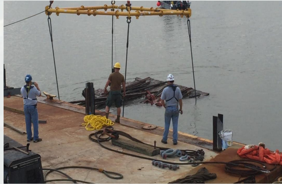
East casemate lift with frame and cables in view
