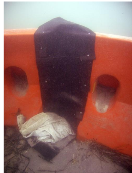
Fig. 3 Plastic damp coursing anchored over the gaps between the RCBs with zinc tek screws. (J. Carpenter)
