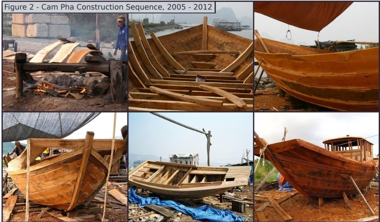
Fig. 2 Cam Pha Construction Sequence, 2005 – 2012. (Ken Preston)
