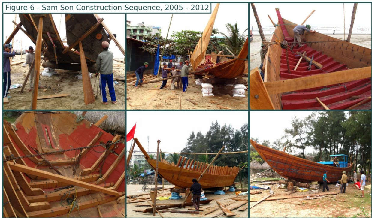
Fig. 6 Sam Son Construction Sequence, 2005 – 2012. (Ken Preston)
