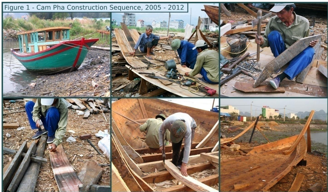
1 Fig. 1 Cam Pha Construction Sequence, 2005 – 2012. (Ken Preston)
