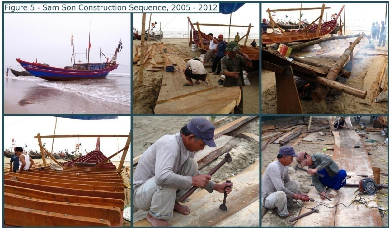
Fig. 5 Sam Son Construction Sequence, 2005 – 2012. (Ken Preston)
